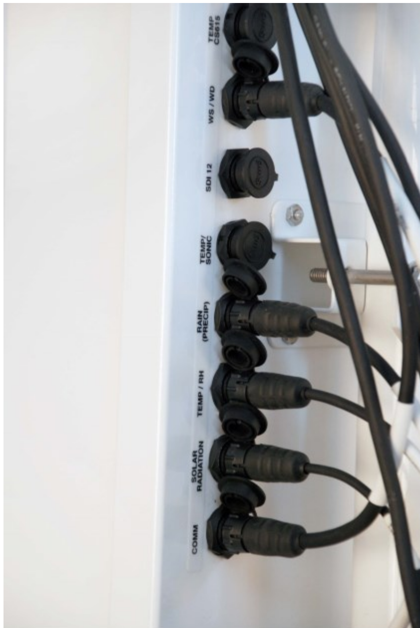
FIGURE 6-21. Connecting sensor cabling to enclosure
